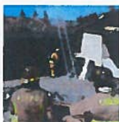
Various San Diego County firefighters train in numerous stages during a burn cadre at the old Fallbrook Golf Course structure. The new owner of the property Jade Work, donated (once approved) the structure to firefighters for training and demolition purposes.
