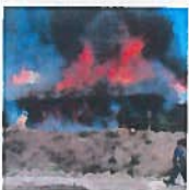
The old Fallbrook Golf Club structure begins to become completely engulfed in flames, March 31.
