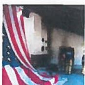
A large American flag hangs inside the Fallbrook Golf Club structure. Firefighters from throughout northern San Diego County participated in a flag retirement ceremony before burning hundreds of American flags in the old structure’s demolition.
