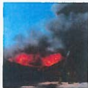
Firefighters wet a large oak tree next to the old Fallbrook Golf Club structure as they let the fire take its course towards demolition of the building, March 31.
