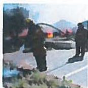
Firefighters put out a small spot fire at the old Fallbrook Golf Club parking lot from wind carried embers as they let the fire take its course towards demolition of the building, March 31.
