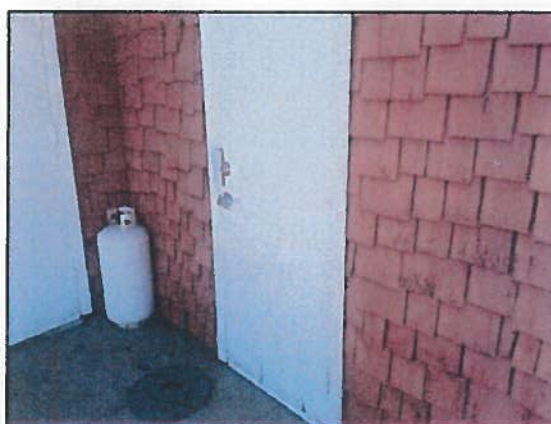
Photo 4 Roy Noon Meeting Hall – Back door swelling and, peeling particularly at base
