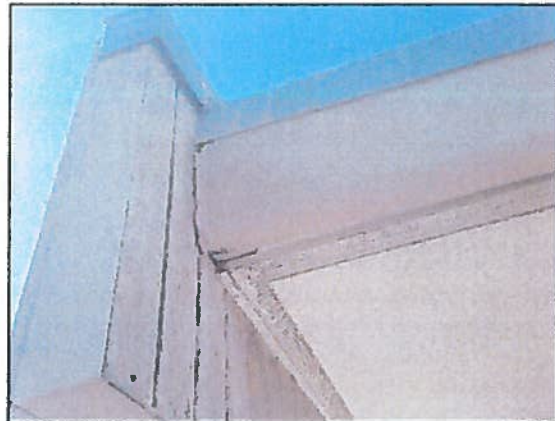
Photo 6 Fire Station 1 – Siding on south side with weathering and mild stucco spalling
