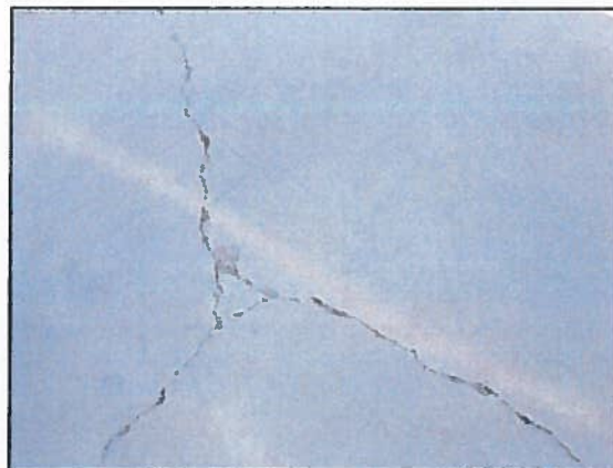
Photo 2 Fire Station 1 – Cracking at driveway/parking area
