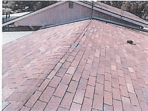
Photo 16 Fire Station 4 – Asphalt shingle roof with worn shingle, loss of aggregate and some missing tabs.
